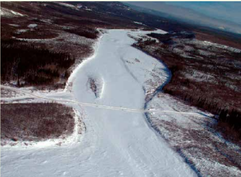
Ice bridge built over large stream channel
