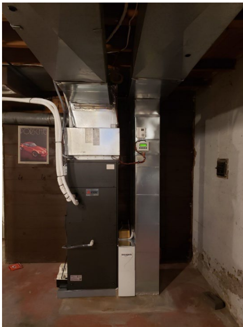
Figure 5 - Central Ducted ccASHPs appear similar to an oil furnace and use similar ducting to circulate hot air around the home
